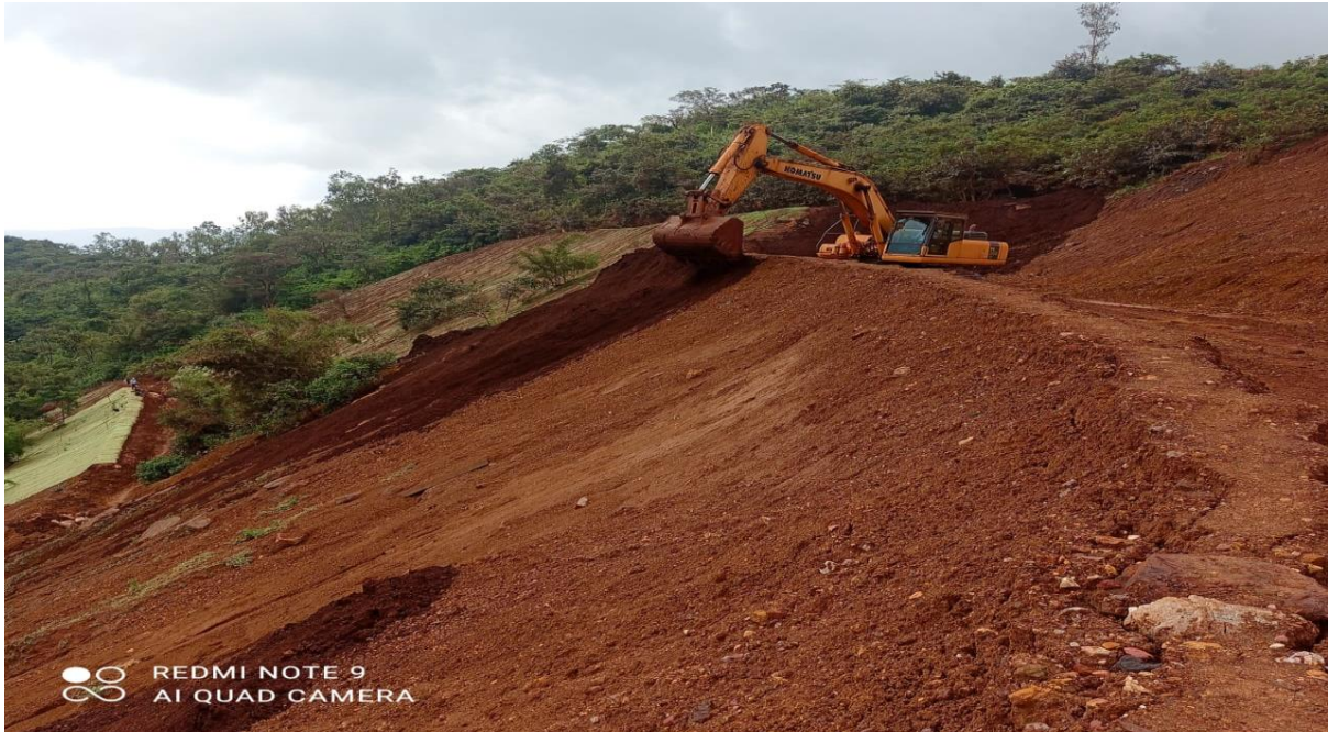
Top soil spreading over waste dump
