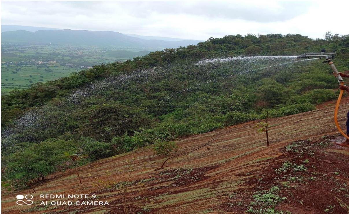
Watering over coir mat set on rejection dump
