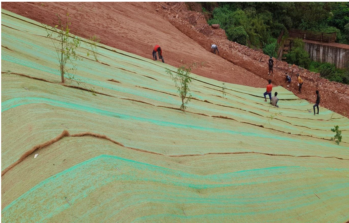
Planting over the Coir Mat and preparing for further coir matting
