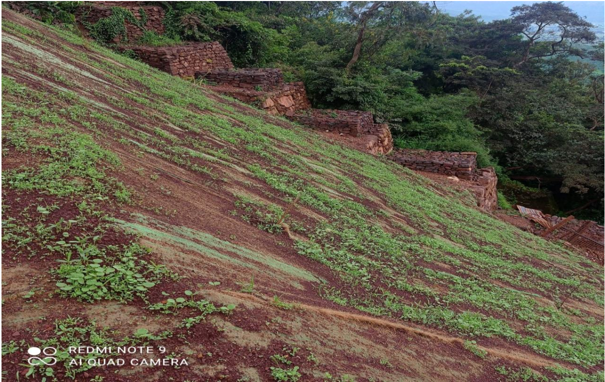
Growth of Grass/Plant seeds over coir mat set on rejection dump (10 days old)
