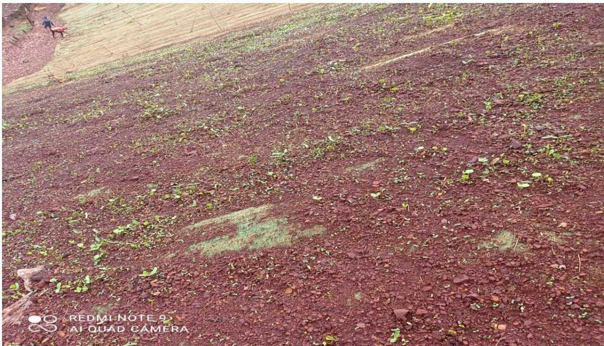
Grass seeds growth over coir mat set on rejection dump(3 days old)
